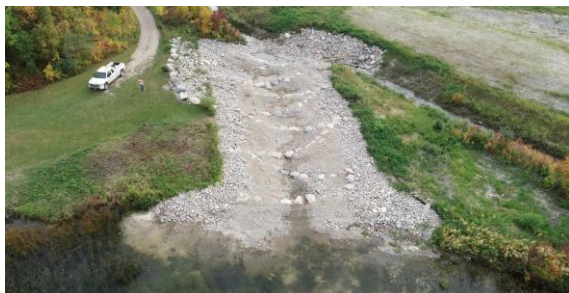
Sand Hill Lake Outlet Rock Arch Rapids Retrofit
