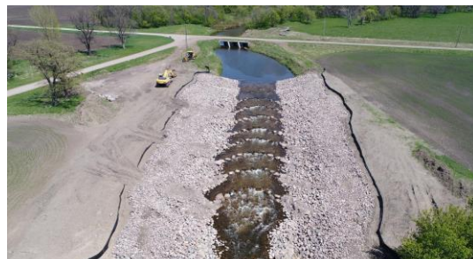
Sand Hill Lake Drop Structure Rock Arch Rapids Retrofit
